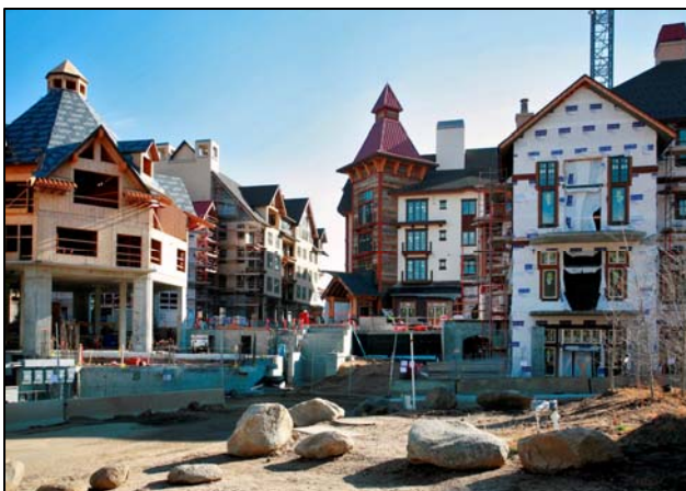
Village Plaza under Construction
